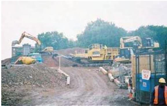
Demolition material is crushed on site for reuse as concrete aggregate or sub-base material, reducing the amount of aggregate to be imported and waste to be exported.
