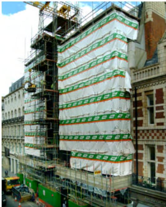
**Figure 7: Building wrapped in monoflex sheeting to prevent escape of dust during construction**
