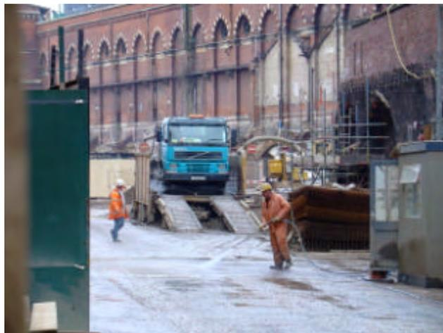
Wheel washing on exit from site reduces nuisance from dust and mud on surrounding roads.
