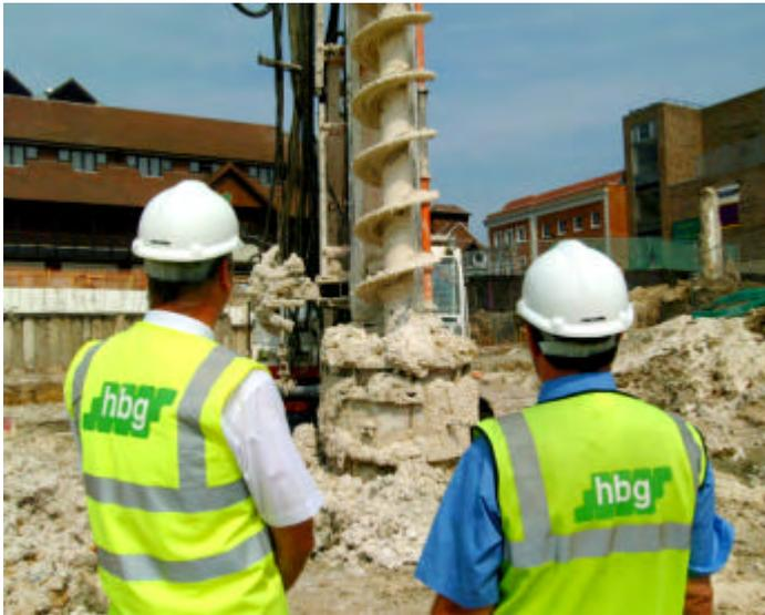
The ground conditions at King's Cross generally suit piled foundations. It is important to choose appropriate methods of piling within an urban environment to avoid excessive noise spilling out into the surroundings. Bored methods of installation (as illustrated) would generally be favoured over driven techniques.
