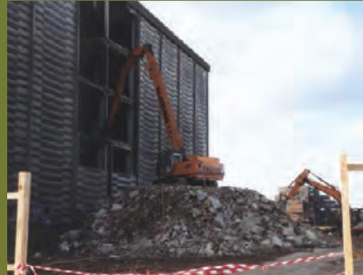
At St George Wharf, Vauxhall St George crushed a disused cold store, generating around 10,000 tons of crushed concrete, which was re-used for temporary roads during construction, and recycled about 2,000 tons of steel.
